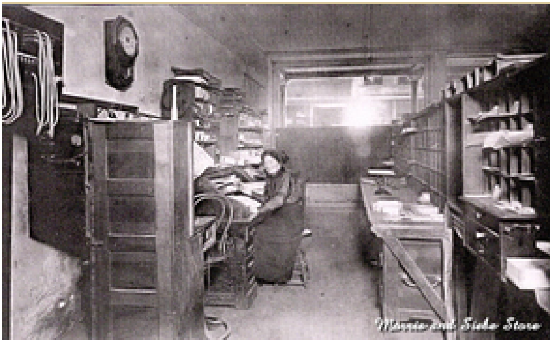
Rose Tam Siebe at her switchboard some time before World War I.
