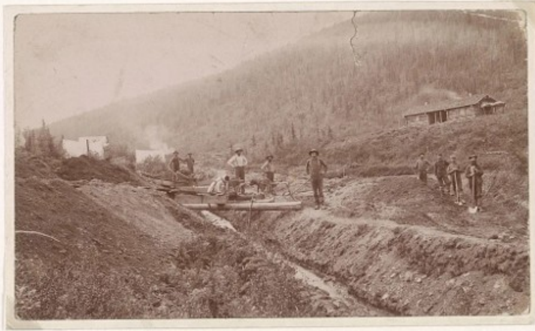
A foothill placer mining operation.
