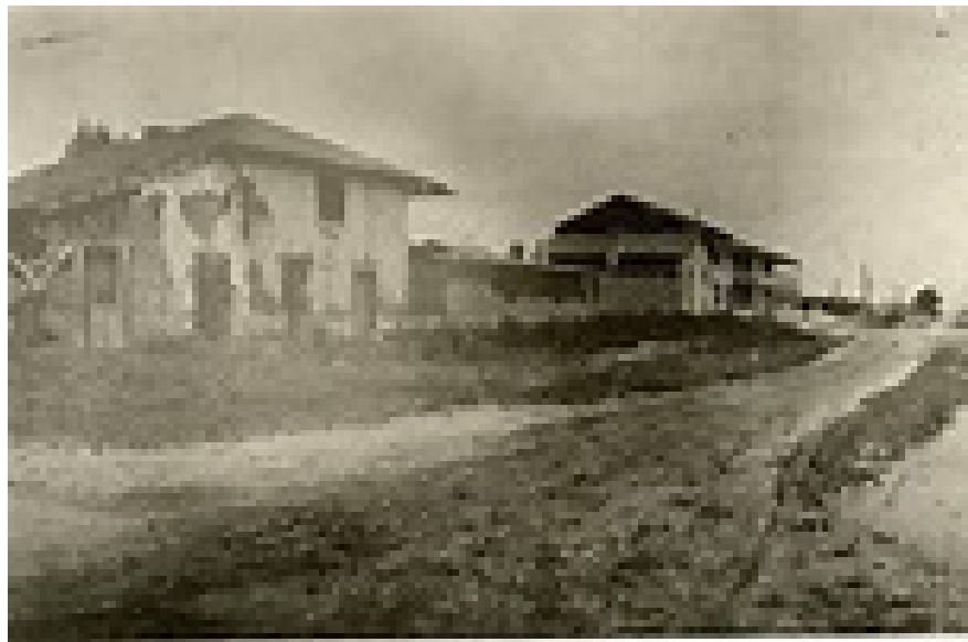
Abandoned buildings from the Mexican period.
