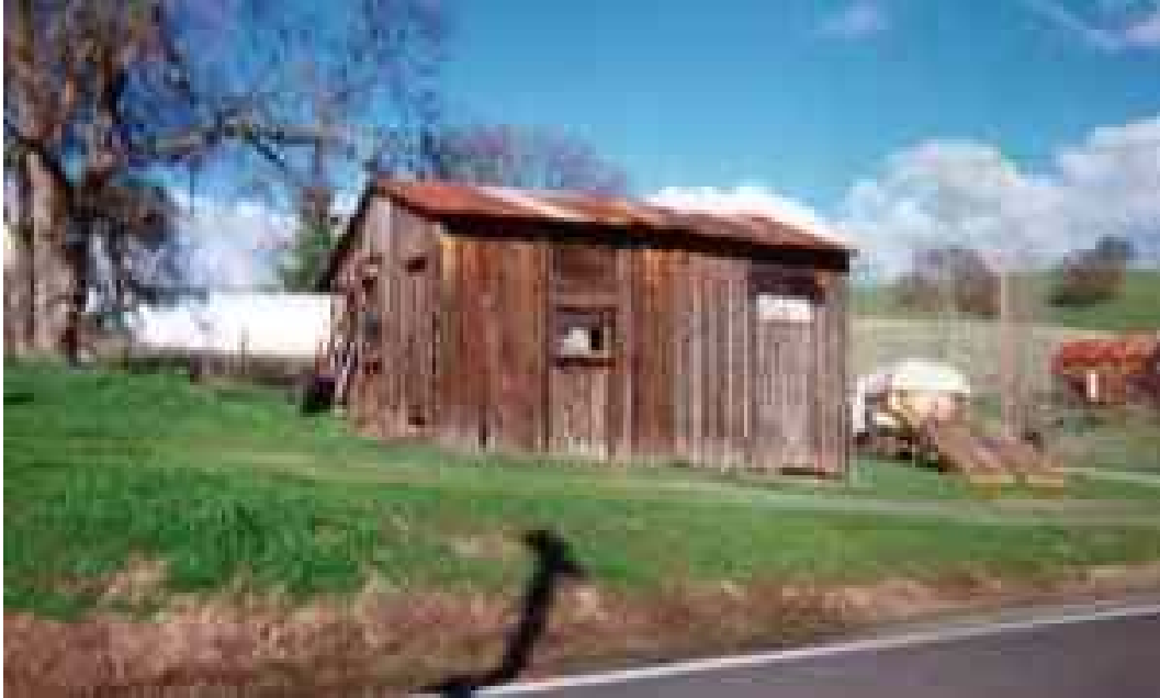
Shack at the site of New Chicago.
