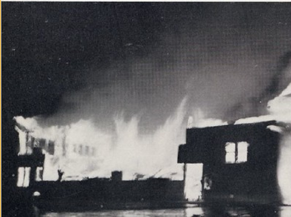
Amador High School Gym set ablaze by wind blown embers on the roof.
