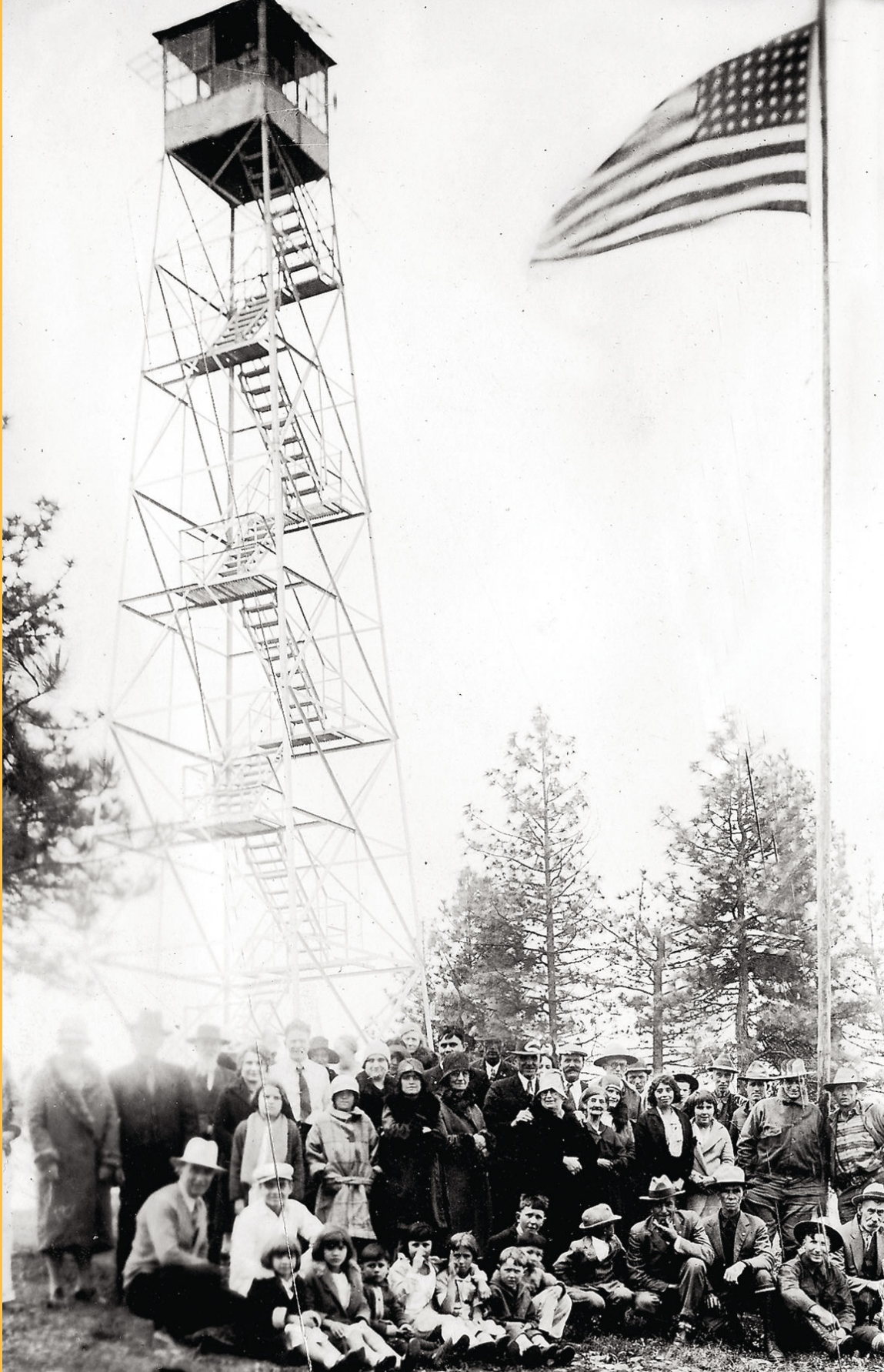
Mount Zion fire look-out tower.
