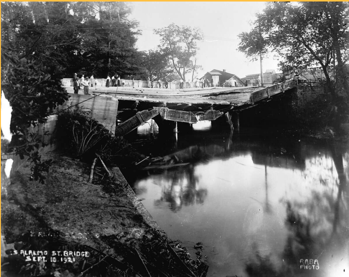
Typical flood damaged bridge.
