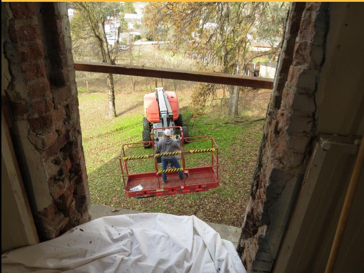
**Once again, the contractors had to custom fit each window into the 150 year old brick walls. The 11 windows on the second floor presented their own set of challenges, such as tapering walls, crumbling mortar, and 2 windows of different sizes with arched tops instead of flat tops.**
